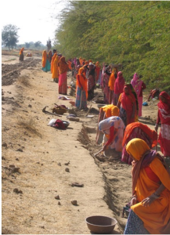
...NREGS road project
